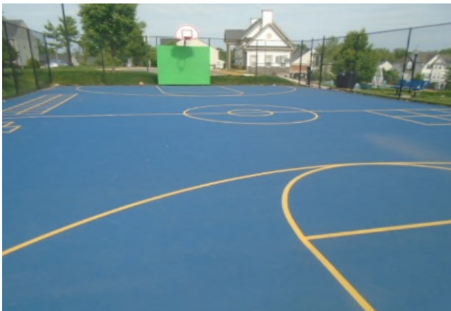
Multi-purpose court was recently color coated. Reserve provides for the next time this work will be needed and rebuilding of the court at end of its useful life.
