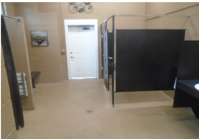
After years of use bathrooms and shower rooms need refurbishing.
